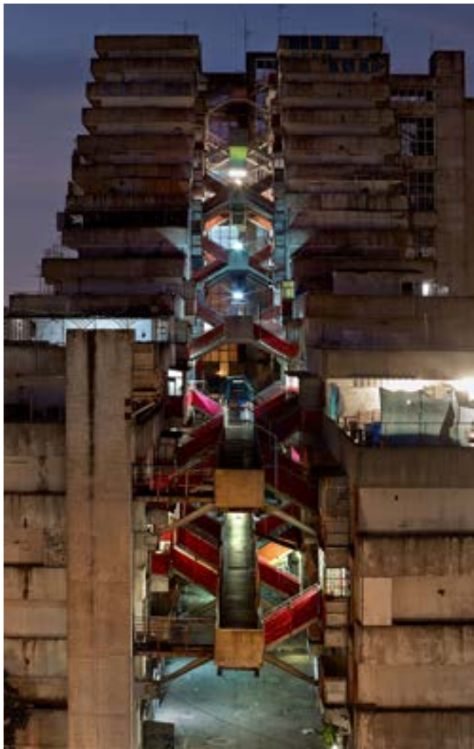
Fig 8. Walkways suspended across void
