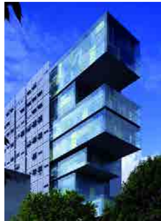
Figure 44. Environmental screen on east façade to protect the interior from over heating (Architect's Journal, 2007)
