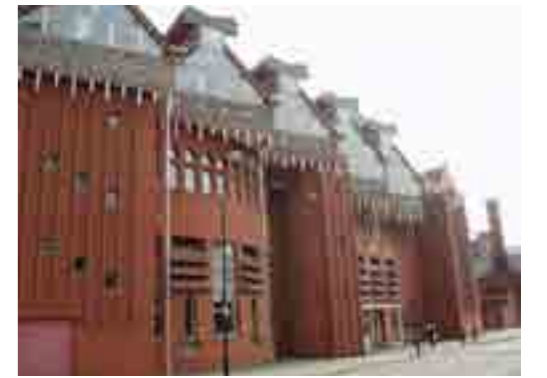
Figure 32. External view of north facade showing louvered inlets that ventilate the auditoria.
