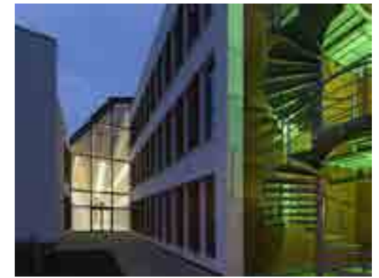
Figure 40. Exterior view of concourse (King, 2009)
